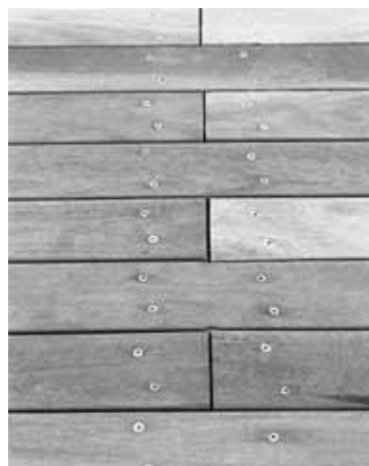
Fig 22 Staggering of plank joins in wide sections of decks is facilitated by paired joists
