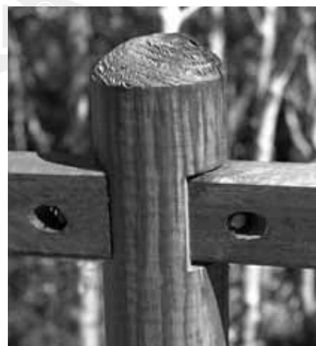
Fig 17 Round handrail post system
