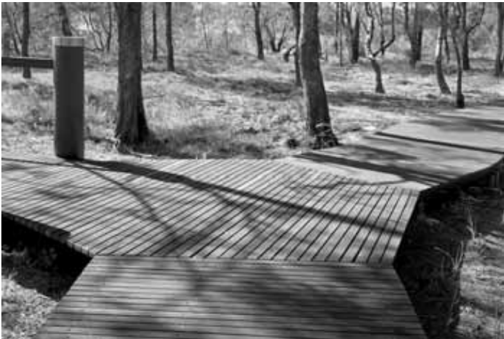
Fig 9 Boardwalk three way junction with truncation
