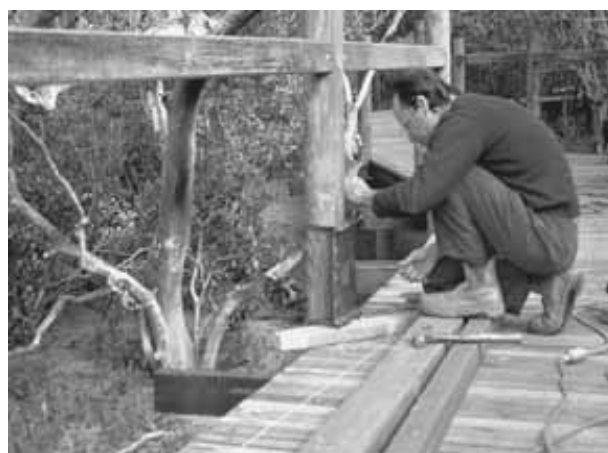
Fig 18 Round handrail post system - router jig
