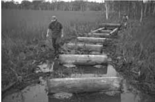
Fig 37 Bedlog installation on poor ground
