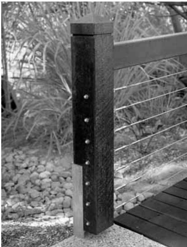
Fig 15 Stainless steel wire as barrier infill.
