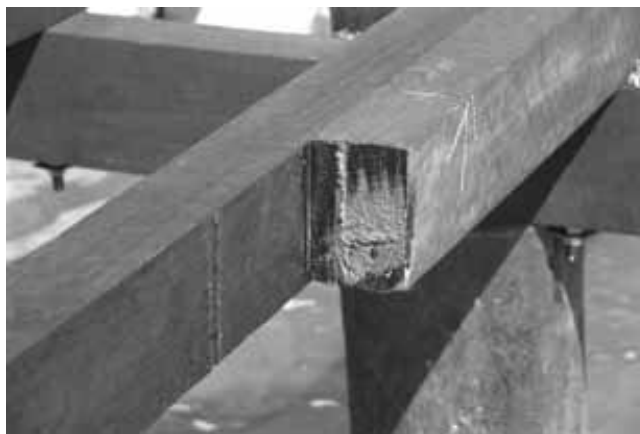
Fig 21 CN Emulsion on cut end
