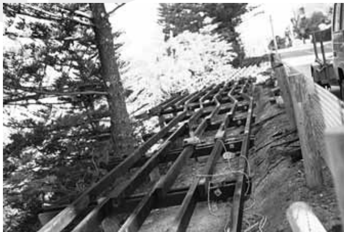
Fig 34 Typical joist framing
