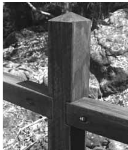
Fig 16 Post projection breaks line of the rail
