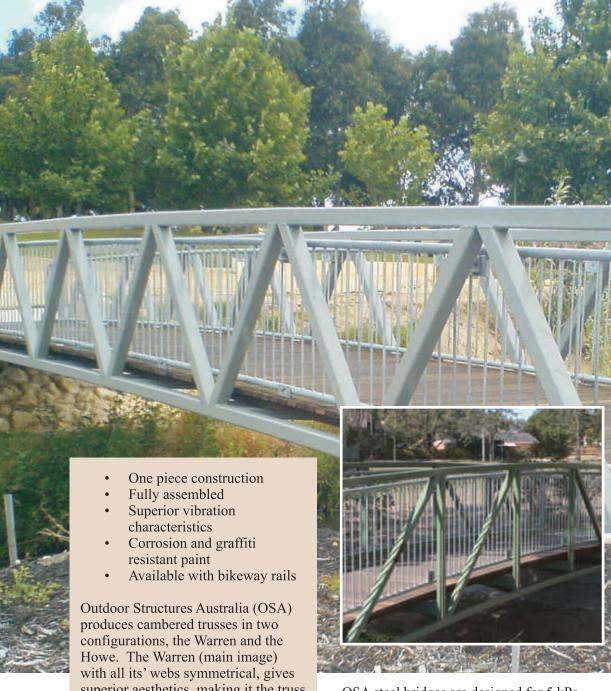
produces cambered trusses in two configurations, the Warren and the Howe. The Warren (main image) with all its' webs symmetrical, gives superior aesthetics, making it the truss of choice for residential subdivisions and high profile locations. The Howe, (smaller image) utilises a vertical web and has slightly better strength characteristics making it ideal for very long spans.
