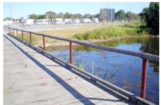
Each handrail has taken a set downward
