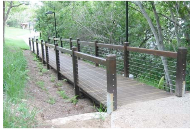
Breaking the line of sight at a posts (rail size 125x75)
