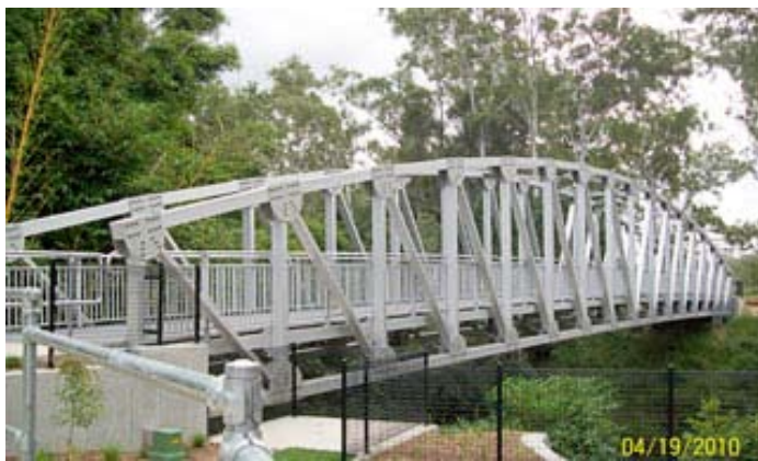
52 metre span Aluminium Bridge, Jindalee
