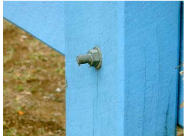
Protruding Bolts are Dangerous
