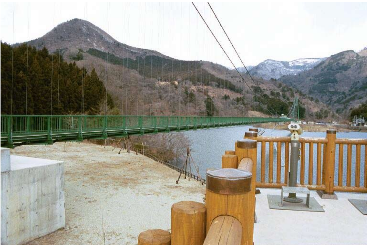
320 metre suspension bridge in Japan with timber decking by OSA
