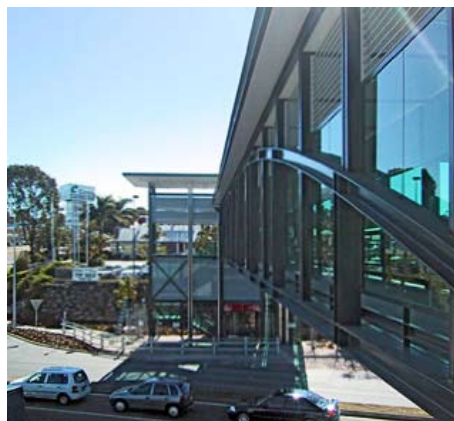
40m span bridge Brisbane
