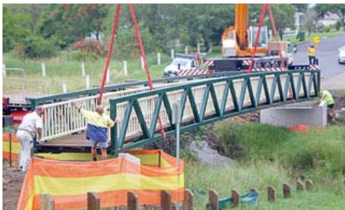
OSA Standard Warren Truss with a 22m span, Ipswich
