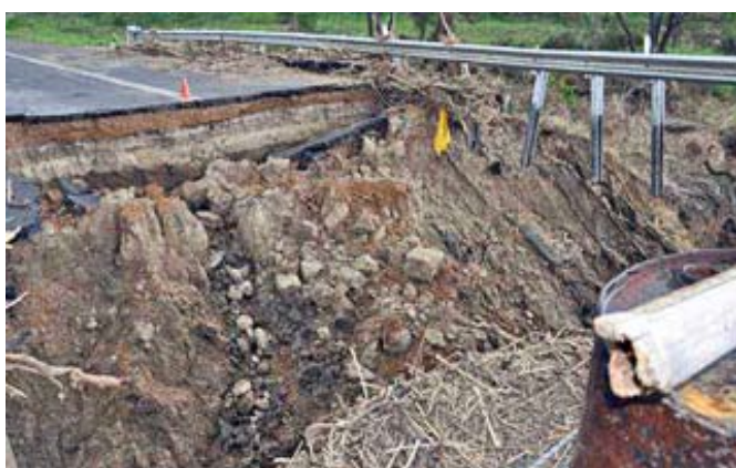
Many bridge approaches had severe washout
