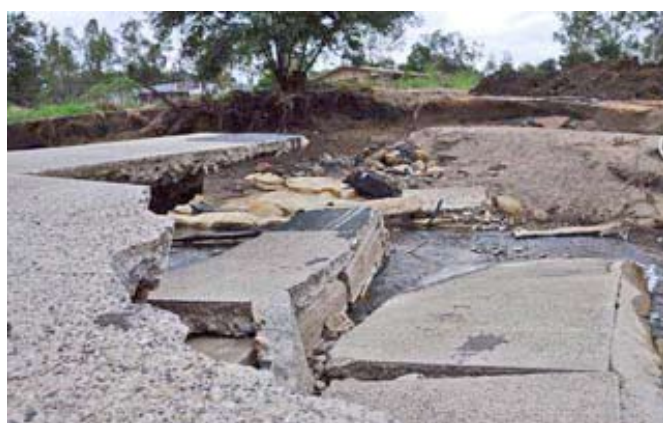
Massive damage to creek crossings
