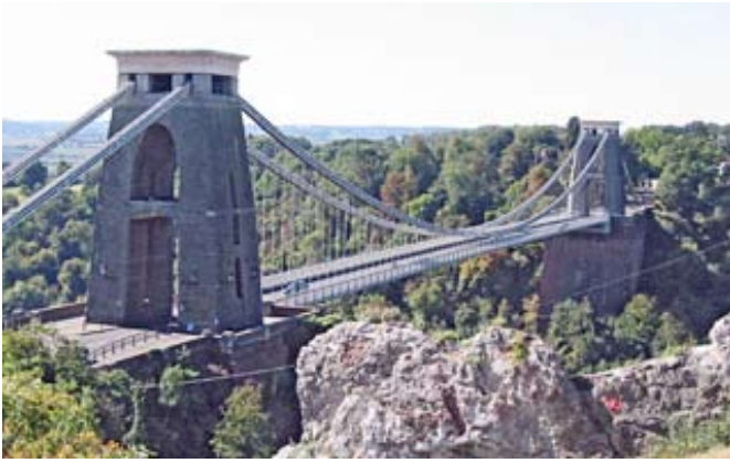
Clifton Bridge near Bristol UK
