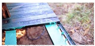
Boardwalk by OSA with Malthoid on top of joists and CN emulsion on top of the Malthoid
