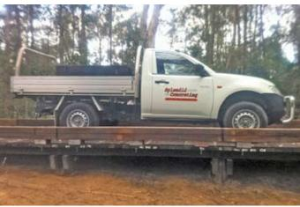
This boardwalk was unusual in that it needed to carry a 2.5tonne, 4 wheel drive fire vehicle. We prepared the drawings for the superstructure based on our standard systems and then emailed the AutoCAD drawing through to the engineer. He checked them and simply dropped the file into his drawings and then designed the site specific superstructure. With OSA preparing the layout the many points of detail we incorporate into our boardwalks were fully detailed.
