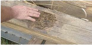
Area around vertical through bolt where Malthoid held water next to the wood bearer causing the cross bearers to decay in 8 years
