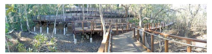
The scope of works comprised two parts. The first, to construct a new access ramp from the lower car park, leading up to the entrance of the wildlife sanctuary. An elevation of approximately 9.5 metres with 153 lineal metres of timber decking and switchbacks.
