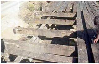
8 year old deck and cross bearers removed due to decay in bearers with Malthoid still showing.
