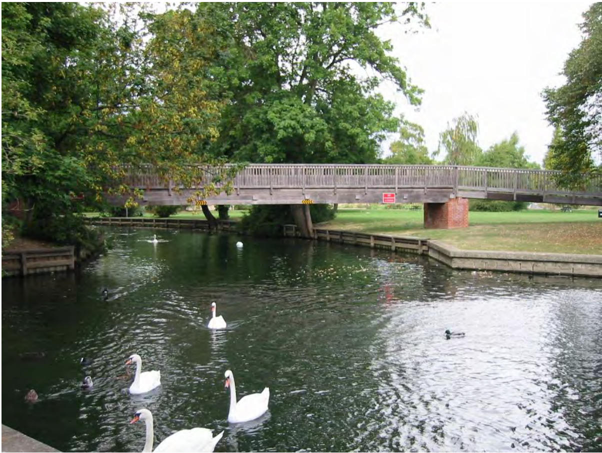
Timber Footbridge at Windsor UK
