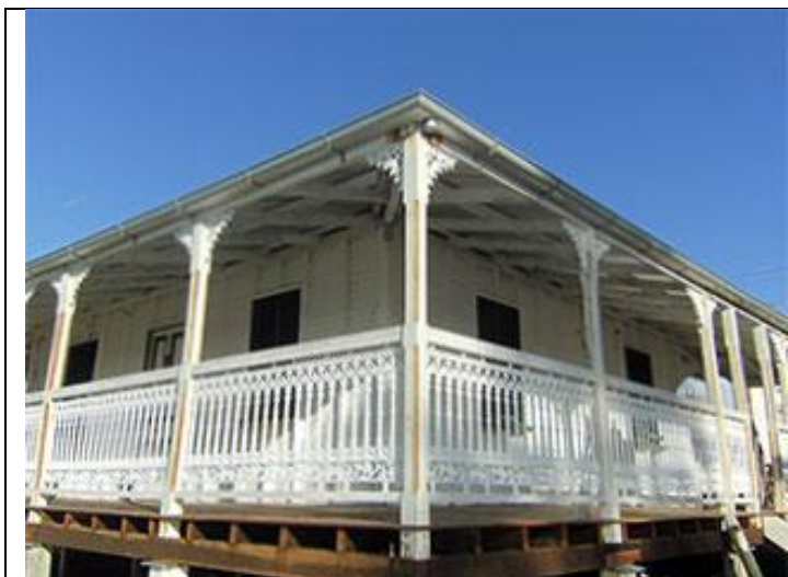
Nonstandard handrail on historical home recreated by Infrastruxion
