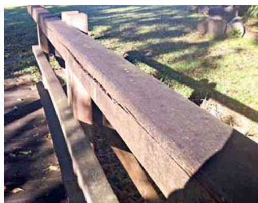
Bridge handrail made from 100x100 heart centre
