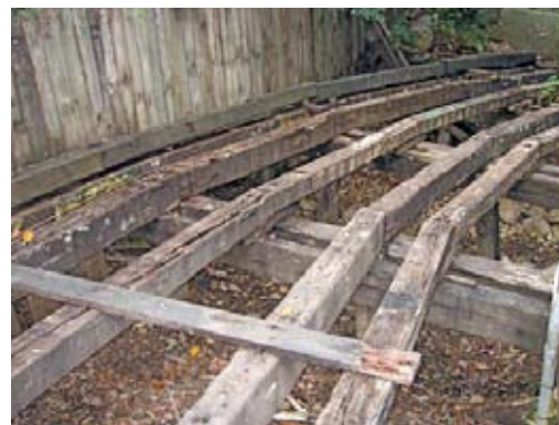
Worn out timber used to construct new access bridge
