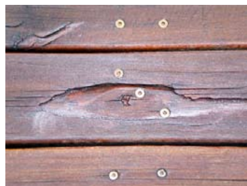
Unsuitable recycled timber used as decking
