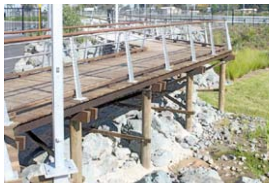
General view of walkway
