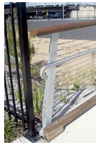
End of handrail
