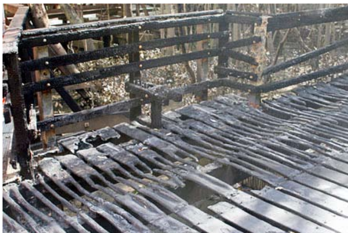
Relatively new plastic boardwalk deck subject to vandalism
