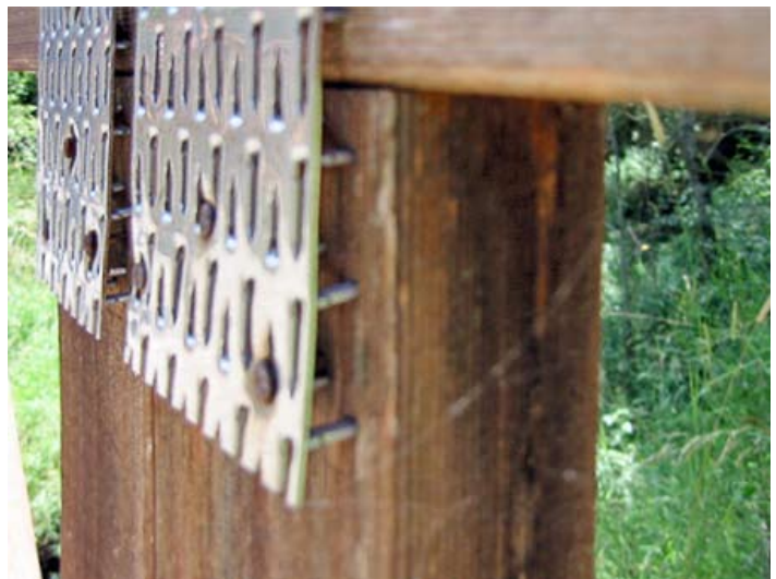
Nailplate virtually falling out of an inexpensive truss bridge
