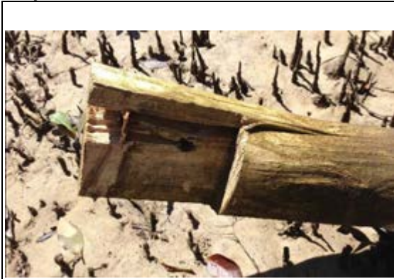
Bolts too close to the post top
