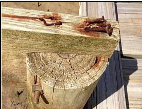
Joists were only nailed on
