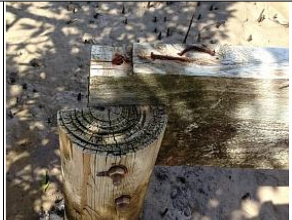
Bolts too close to the borer end
