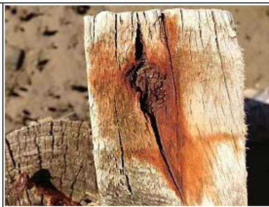
Rusting nails have damaged the timber
