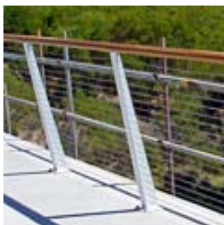
C4 Cycleway barrier system
