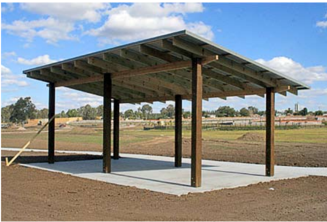
Copy of an OSA Lindsay 10x4 shelter when first installed
