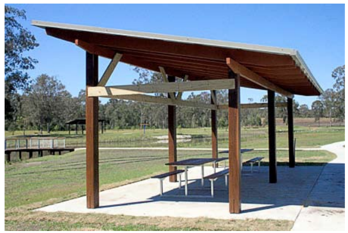
Extra bracing later added to the shelter to stop it shaking
