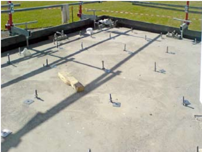
Support studs for joists
