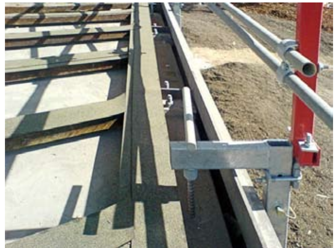
Joists ready for Decking
