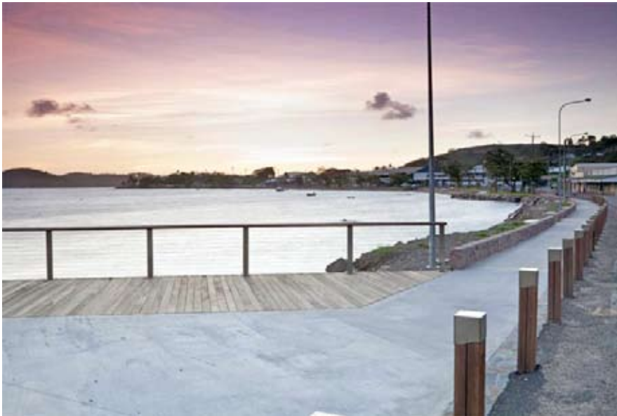
Thursday Island Foreshore deck and bollards
