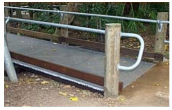
Termination uses iron bark joist NOTE Caps were not Installed when these images were taken.
