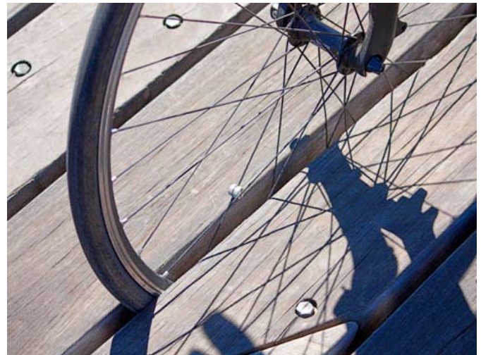
One of our readers was injured by this 29mm gap
