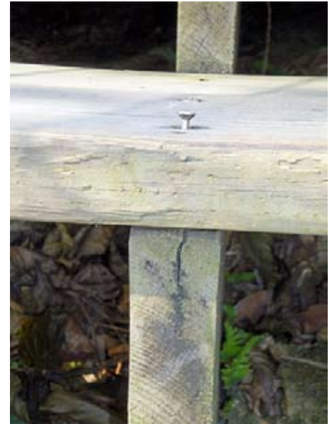
Protruding Screw is very dangerous
