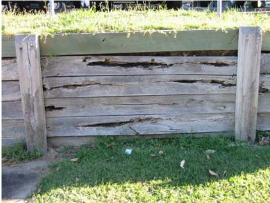
This sleeper wall used timber of low quality which is deterioration quickly. One whaler has already been replaced. This retaining wall would not have been designed using this grade of timber. The sleepers would have been supplied on the basis of price, not specification
