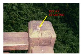
The post on the left is 150x150 with the heart in the centre. Because the heart is much softer than the surrounding true wood, the centre decays as the image shows. A metal cap protects this soft timber from decay and also restrains the top and helps minimise the splitting. The cap on the right, a standard OSA product, is smaller than the post as it is designed to allow for a sawing tolerance of +9mm or -3mm for sizes 200mm and over. (sizes under 200mm have a tolerance of + or -3mm.
