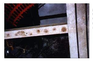
The decking was installed on this joist following the instructions in our Boardwalk Construction Guide at the time (prior to the addition of malthoid). After **two years** there is still no splitting of the joist associated with the screw fixings. The use of malthoid dampcourse reinforces the effects of good practice.
