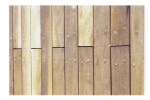
This image shows decking joined on a double joist, The screws are a good distance from the end so there is no splitting of the decking. There is no damage to the joist by having too many fasteners. Note that the boards to not touch that ensures moisture is not held against the end grain by capillary action.
