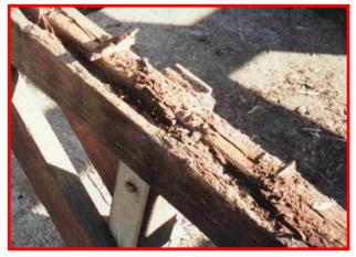
Careful attention must to be given to detailing the joist to ensure that after the decking has served its useful life, the substructure is still structurally sound and does not need to be replaced as well.
