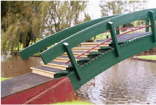
In our guide we refer to the maximum rise for a bridge being 1 in 8. That does not mean that if the bridge is 8.0 metres long the rise in the centre is 1.0m. The measurement is taken from a tangent at the beginning of the bridge where the rise is steeper. The image shows how this rise is not equal over the length. The introduction of stairs into a public structure like this would now be unthinkable, as everything in Australia has to be designed
