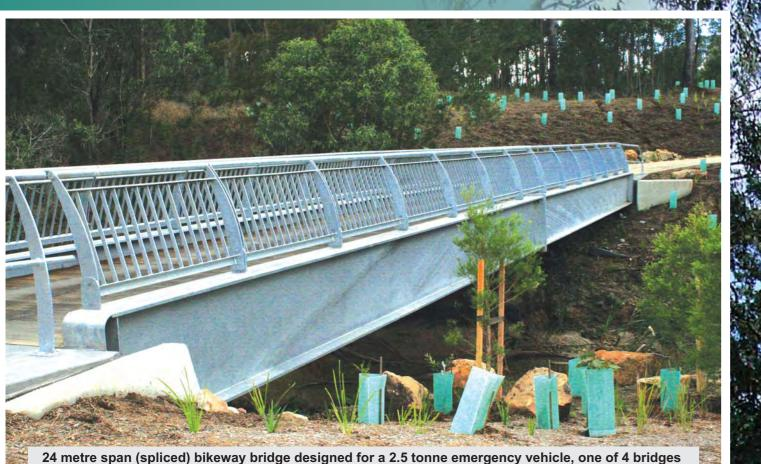
24 metre span (spliced) bikeway bridge designed for a 2.5 tonne emergency vehicle, one of 4 bridges of similar style. Other spans were 12 + 18 m. Designed for flood loading.
