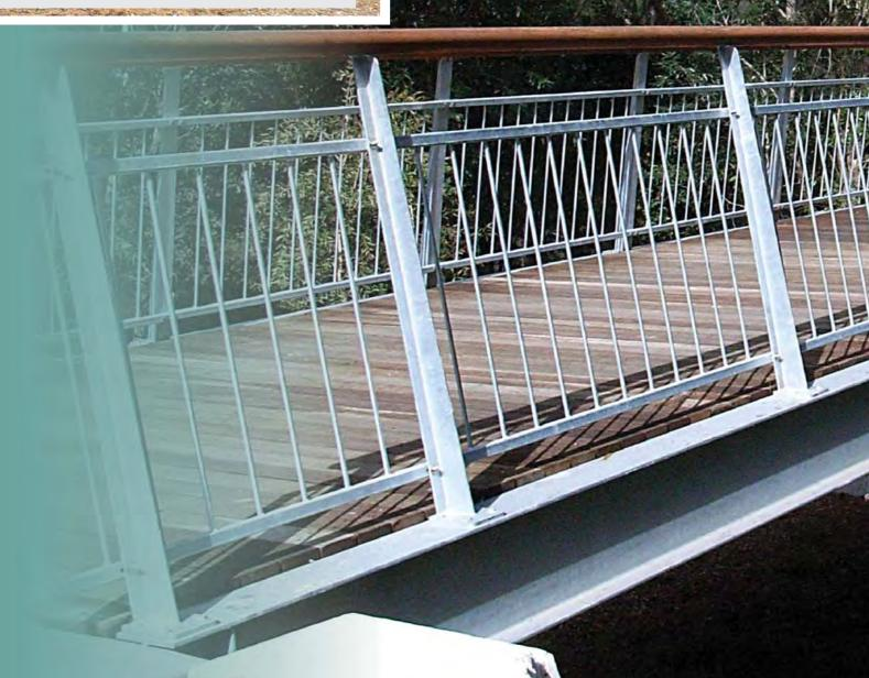
6 metre span swale drain bridge designed for pedestrian traffic. One of 2 bridges of a similar style.
