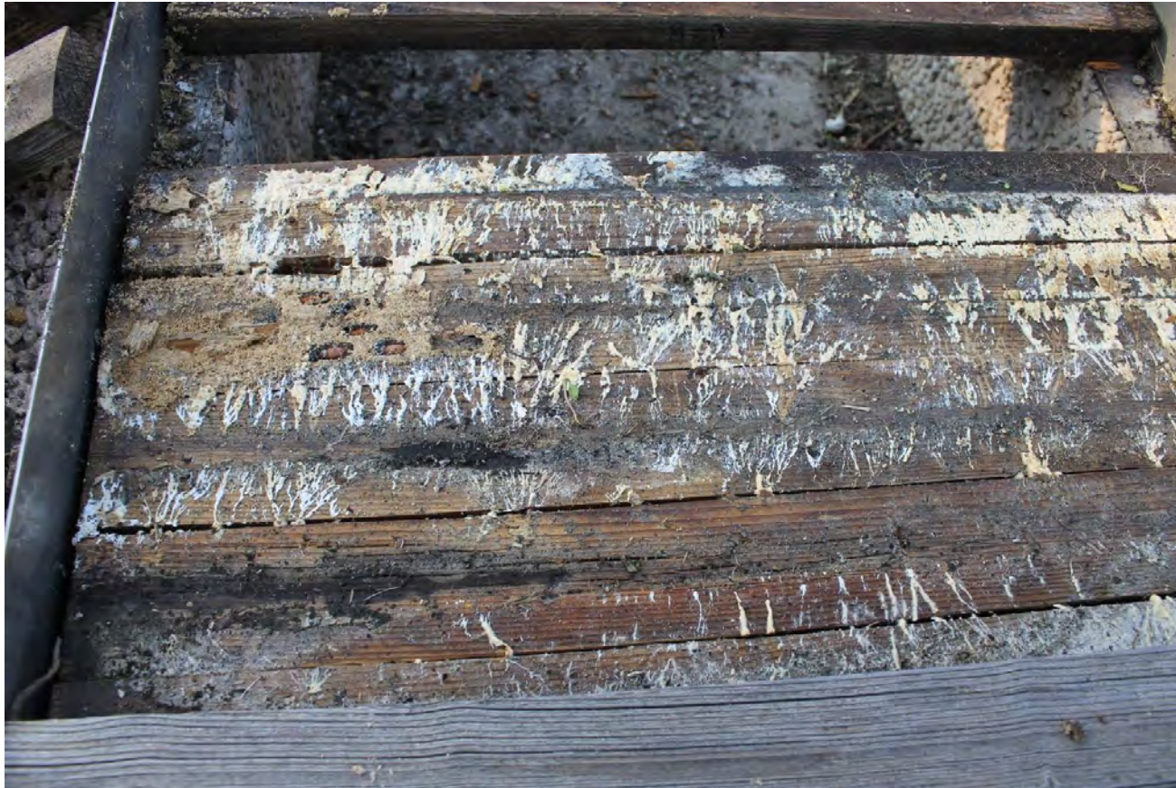
Severe decay or failure due to decay
