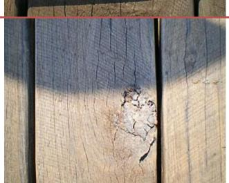
Unsound Knot, Treat as knots as in the table above. There is a pocket of resin associated with a knot. Over time the resin will degrade and wash out and leave a trap for heels
