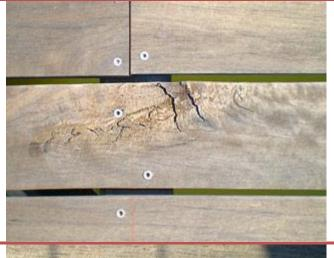
Cross shake (fracture) in conjunction with a knot. Fractures are not permitted at all under AS2082 .This defect covers over half of the board. Again this meets no F rating.
