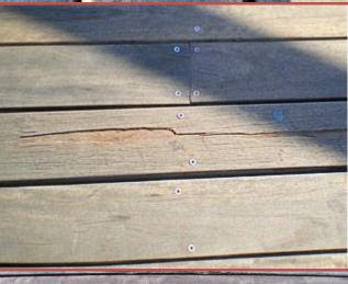
Shelling Out. Shelling out occurs when there is delamination between the growth rings. These have sharp splinters that have to be made safe as soon as they are seen. This example of delamination, which is going across the boards was evident at the time of production and should have been docked out
