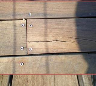
End Split Associated with Heart. This is a hard one for the uninitiated. Notice how the timber down the split is a lighter colour and there is a small knot in it. This is characteristic of heart. AS2082 forbids any heart at all but in reality the decking can carry a touch on the back. But definitely none on the front.
