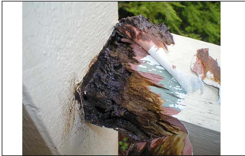
Decay of incorrectly installed LOSP pine handrail
