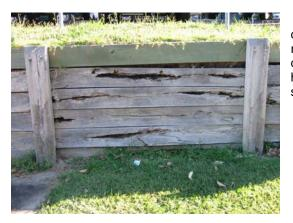
This sleeper wall used timber of low quality which is deterioration quickly. One whaler has already been replaced. This retaining wall would not have been designed using this grade of timber. The sleepers would have been supplied on the basis of price, not specification
